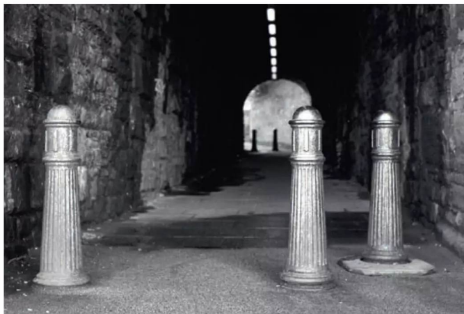
Bollards guard the entrance to a long and gloomy foot tunnel
