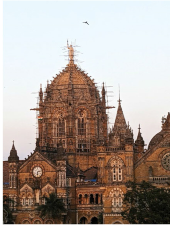
CSMT building undergoing repairs
