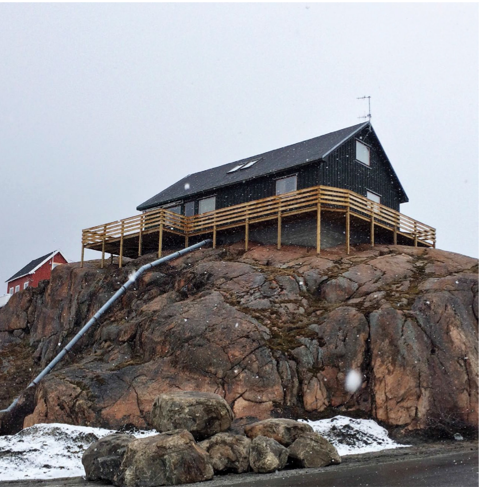
Since large parts of Greenland experience permafrost, houses are built on top of rocks to provide a stable foundation and also for better insulation and protection.
