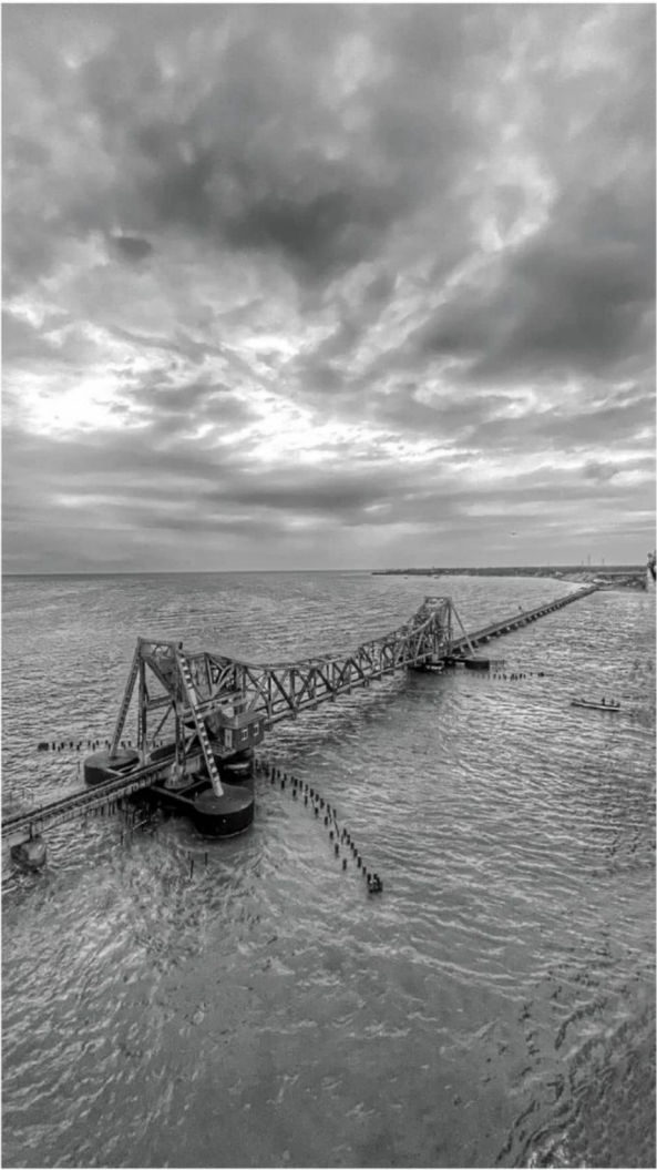
Completed in 1914, the old Pamban Bridge uses a 65-metre lift span weighing about 115 tonnes. Its simple truss-and-lift design shows how engineers solved rail connectivity to Rameswaram in a harsh marine setting in the Indian Ocean.
