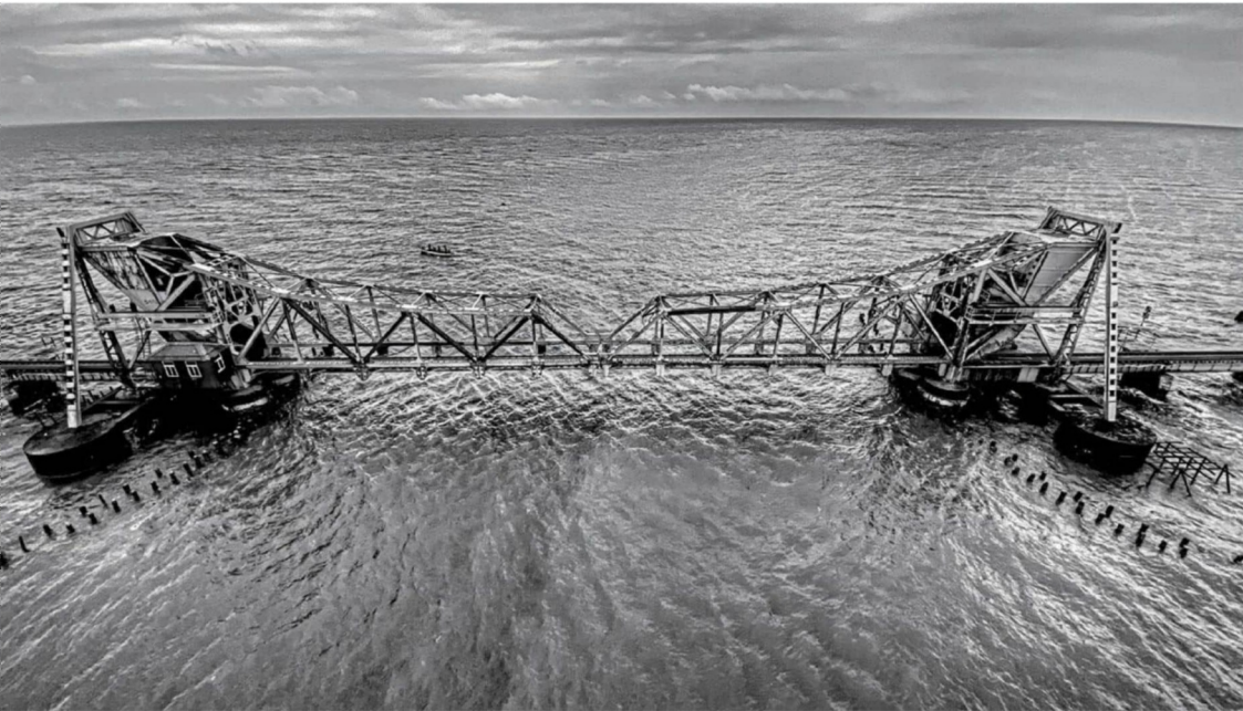
The old Pamban railway bridge, opened in 1914, was India's first sea bridge and remained the longest until 2010. Its iconic double-leaf bascule allowed ships to pass, making it an engineering marvel of its time.
